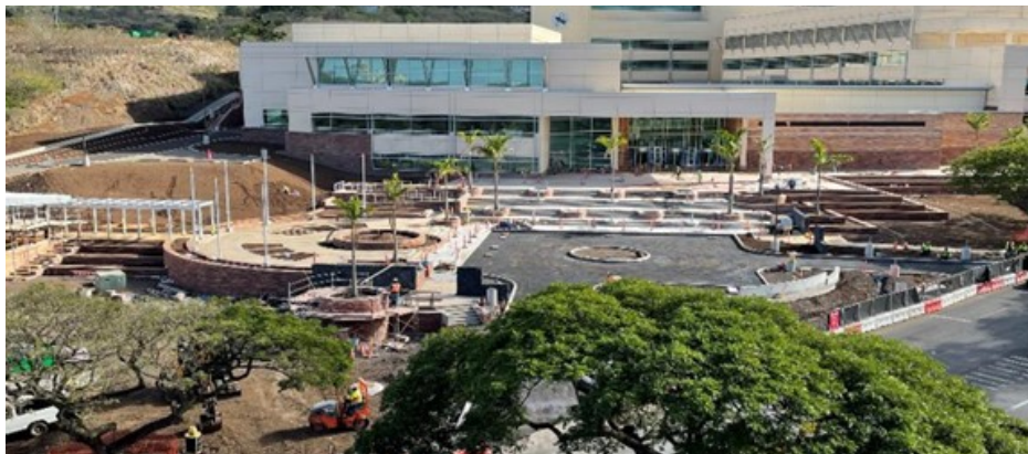
USARPAC Command and Control Facility Fort Shafter, HI
